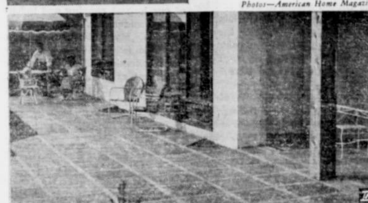
The terrace, above, is made from a form made of sixteen 22-inch squares. No extra preparation of ground is required. Squares are filled with concrete colored with plaster colors to individual taste. Described in detail in the March issue of American Home Magazine, it costs 8 cents a square foot, and a minimum of work to complete.
