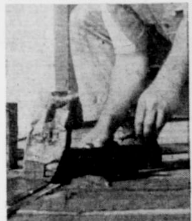
Greased form, set on levelled ground, is filled with concrete.
