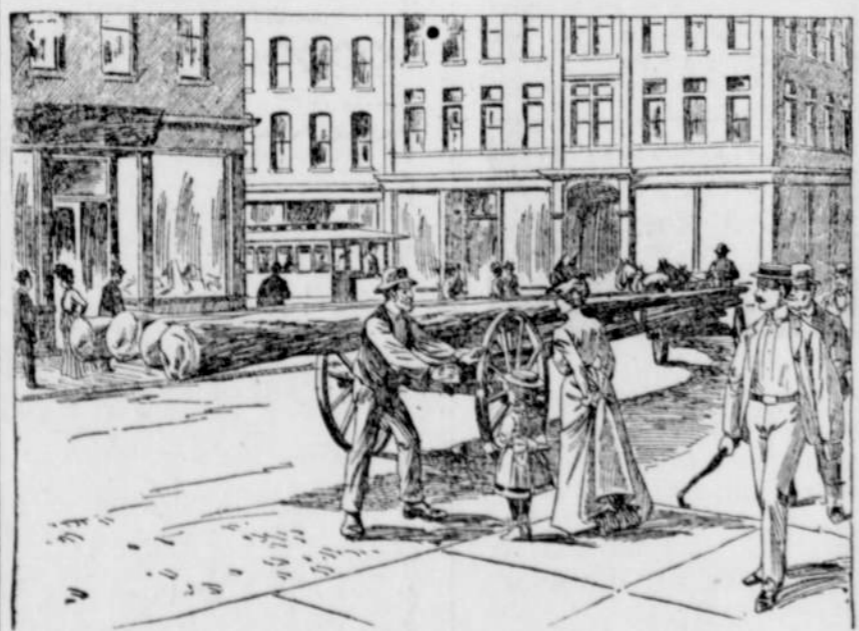
PILOTING LONG POLES THROUGH THE STREETS.
