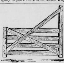
PROPERLY CONSTRUCTED GATE. a gate should sag if it is properly constructed. A proper construction is shown
