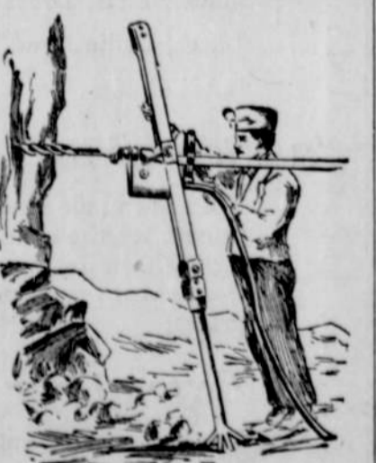
BORES A SIX-FOOT HOLE IN A MINUTE.
