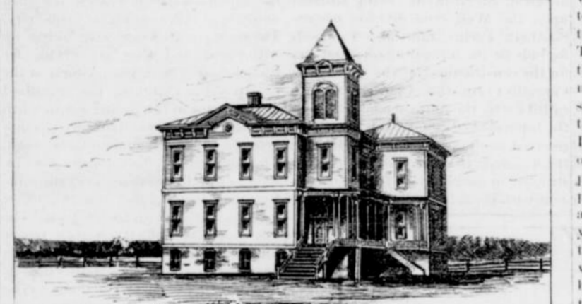
PUBLIC SCHOOL BUILDING, McMINNVILLE, OREGON.
