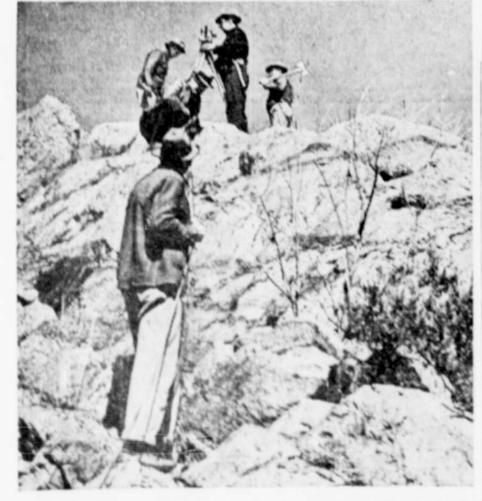
On mountain peaks general land office surveyors obtain scientific measurements to insure accuracy in the new official master map of the United States. As the transit man places his instrument in position, linesmen stretch the steel tape along the correct line into the valley.
