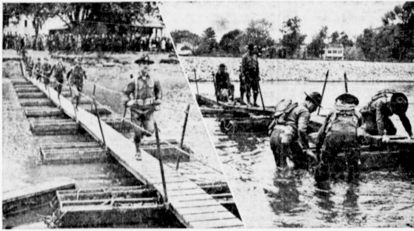
Rapid assembly of a footbridge across the channel of the Chesapeake and Delaware canal was demonstrated at Delaware City, Del., recently at the annual reunion of the First Engineers, U. S. army. Right: Army engineers assembling the footbridge, the work being completed in eight minutes. Left: Army troops as they advance over the footbridge.
