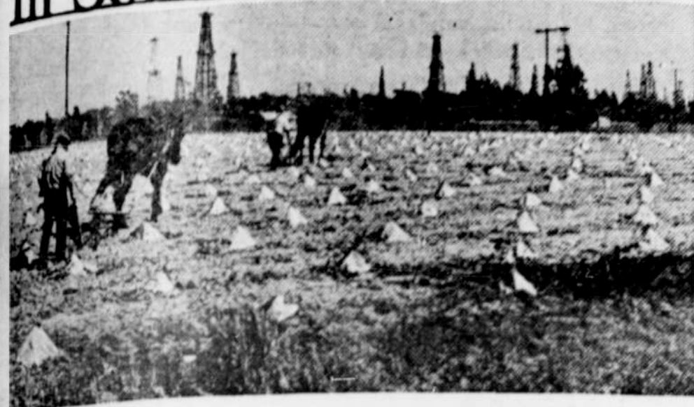
Oil Derricks Form Background for Tomato Patch.
