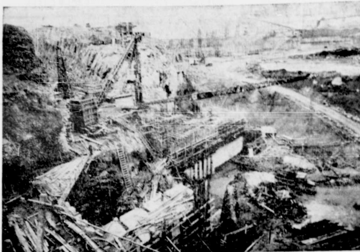
General-Shea men are rushing work on the up-river end of the deep-sea locks, pouring concrete to the 36-foot level so as to form a protective barrier between the powerhouse and the locks. The latter must be kept dry during the high-water, and the huge concrete slabs will have to be in place before the government's tentative safety date, April 15.
