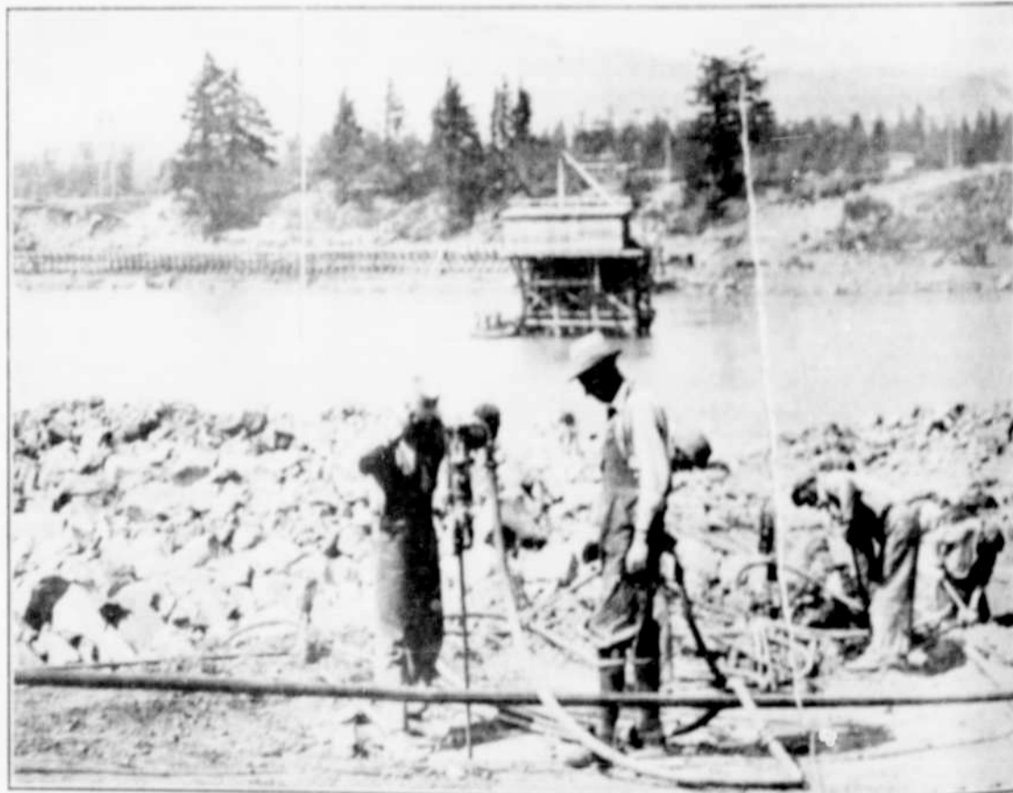
Model S. 55 drill in action at Bonneville on center line of main dam.
