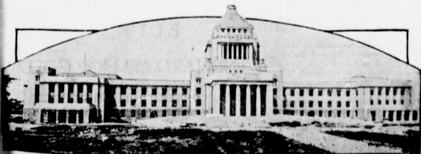
This handsome building in Tokyo, the new houses of parliament, is nearing completion. It is of Japanese design and construction throughout, the only foreign articles being a mail chute and a thermostat.
