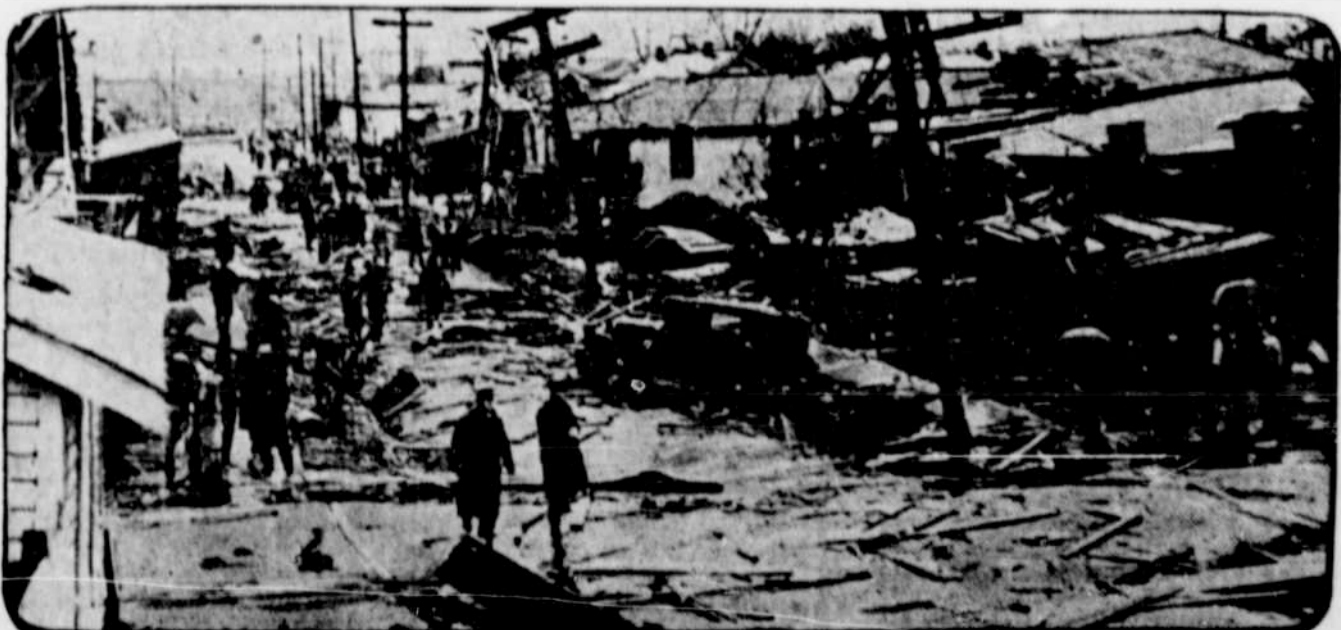
A general view looking down Eads street, New Orleans, showing the damage wrought by a wind storm. One hundred homes were demolished.
