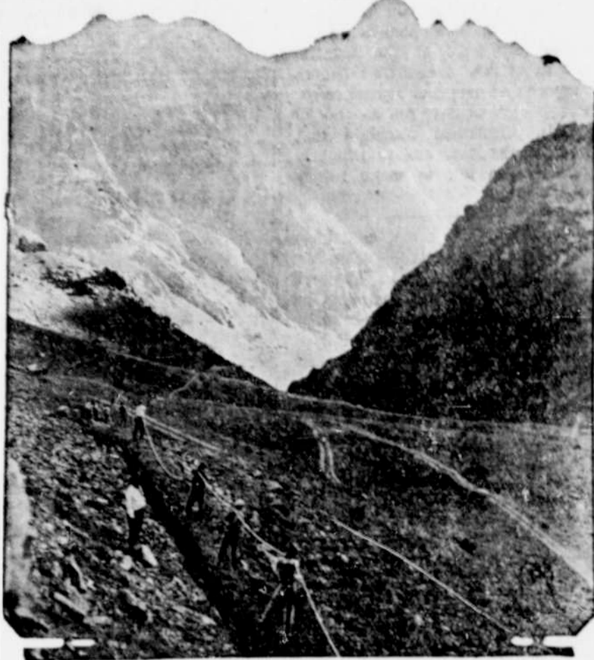
Laying the Trans-Andean Cable.
