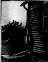
inderground tank provided with tight curb. The filter is filled with layers of charcoal, sand, and screened gravel of small size which have been placed in the container in the order named. The water which comes from this "well" is highly colored but it is exceedingly cold and palatable. From a sanitary standpoint it is perfectly healthful. Before this means of procuring water for drinking purposes
