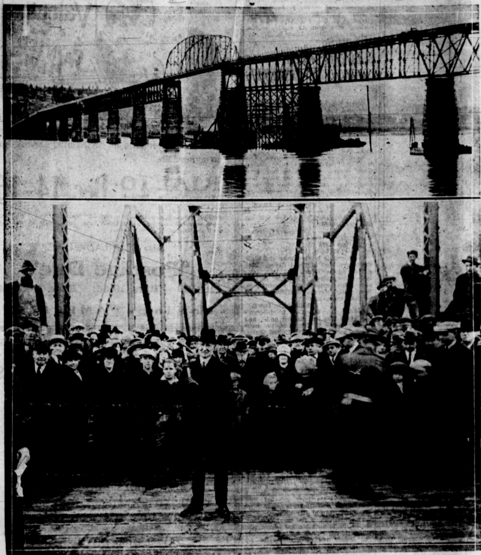
Above—New span with hills of Hood River in background. Below—Leslie Butler driving the last spike. Photo by Reeves.
