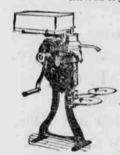
The only separator that starts the easy way,-by "pumping." This manner of speeding up is made possible by the quick catching and releasing clutch.
