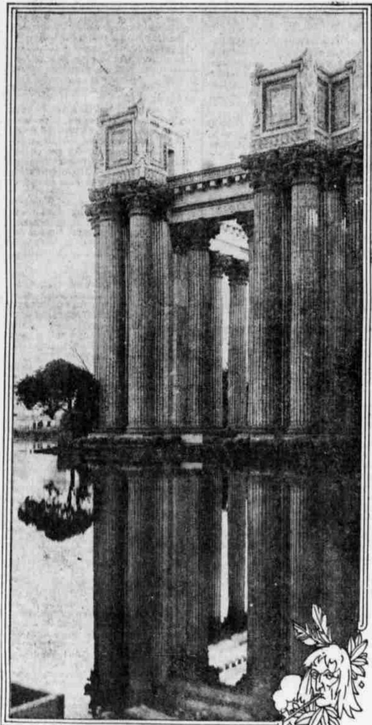
Curving 1,100 feet around the foliaged shores of the Fine Arts lagoon, Panama-Pacific International Exposition, these mighty pillars are reflected, mirrored, in the limpid waters of the lagoon, affording one of the prettiest views at San Francisco's great Exposition.
