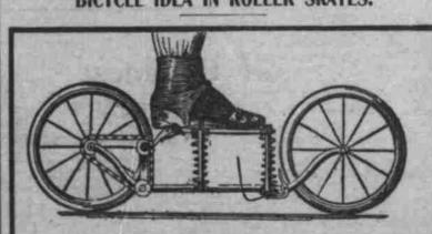
Here is a roller skate that is a sort of blevele for the foot. It has only just been patented. The weight of the skater resting upon one foot pushes down a spring, which is so arranged by gearing with the rear wheel as to propel the whole mechanism powerfully. The skater need hardly do more than walk along, and the machine does the rest, pushing him ahead at a tremendous speed.
