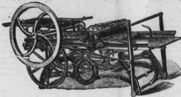
a Prouty press, or, as it is sometimes called, a "Kansas Grasshopper." It is an ideal press for a country office, as it can be run by hand or power at a speed of 800 per hour, and will take a 6-column quarto if special chases with steel side and foot sticks are used.
