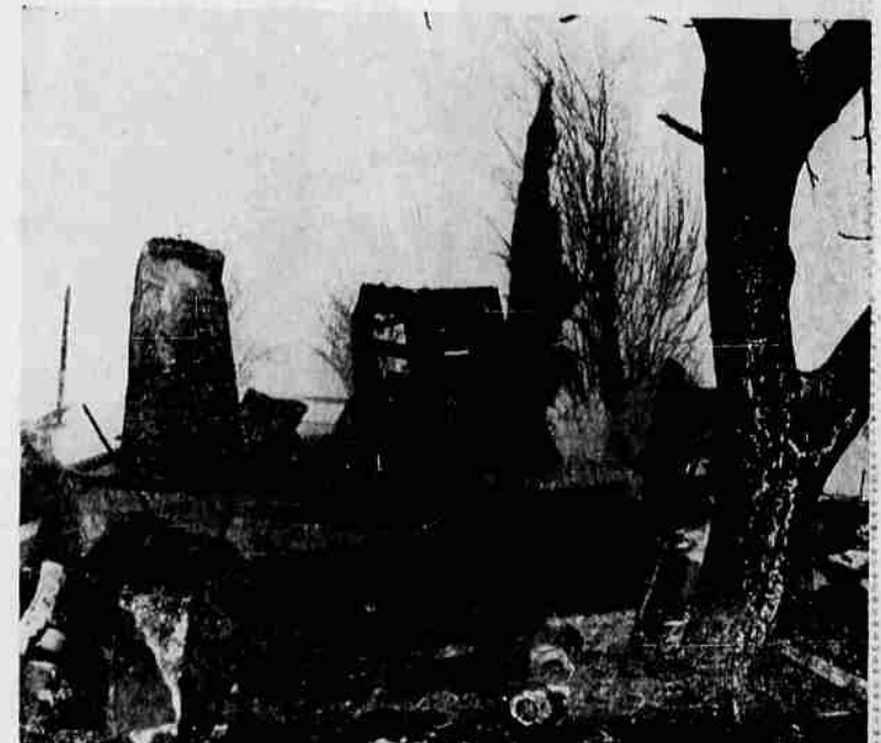
Radio Station KDOV was leveled by fire, one of the major ones in Medford during 1963.
