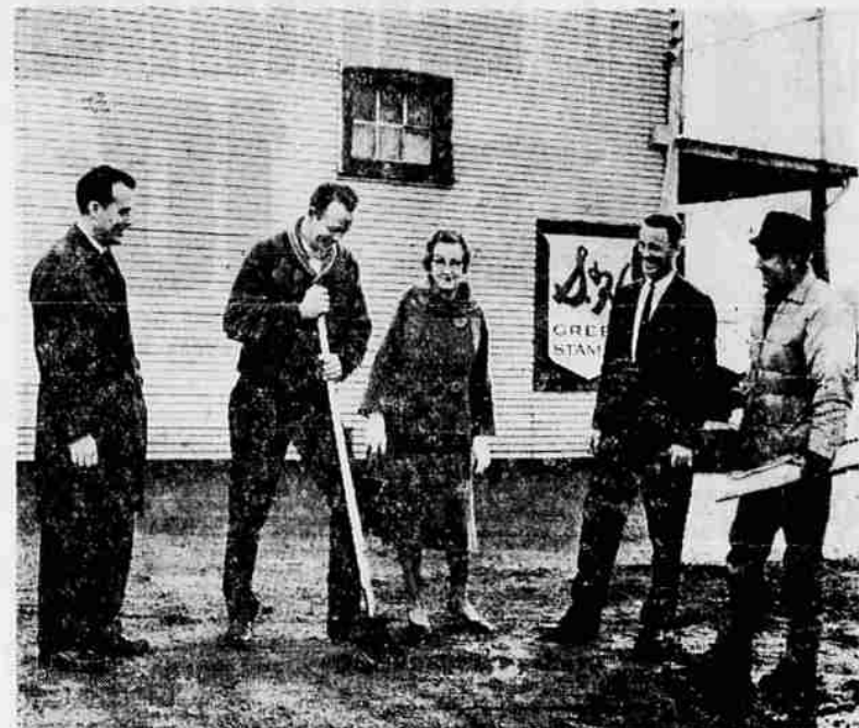
AT GROUND BREAKING — Harold Ellis is shown breaking ground for construction of a 27-unit apartment, Ellis Manor, at the corner of Crater Lake Avenue and Spring Street. Left to right are Rollin Watson, assistant vice president of Equitable Savings and Loan; Ellis, his mother, Mrs. Ellis, part-owner and manager; Kenneth McHugh, manager of McHugh Plumbing; and Donald Kahl, representing Kahl and Johnson Construction Co., which will build the structure.
