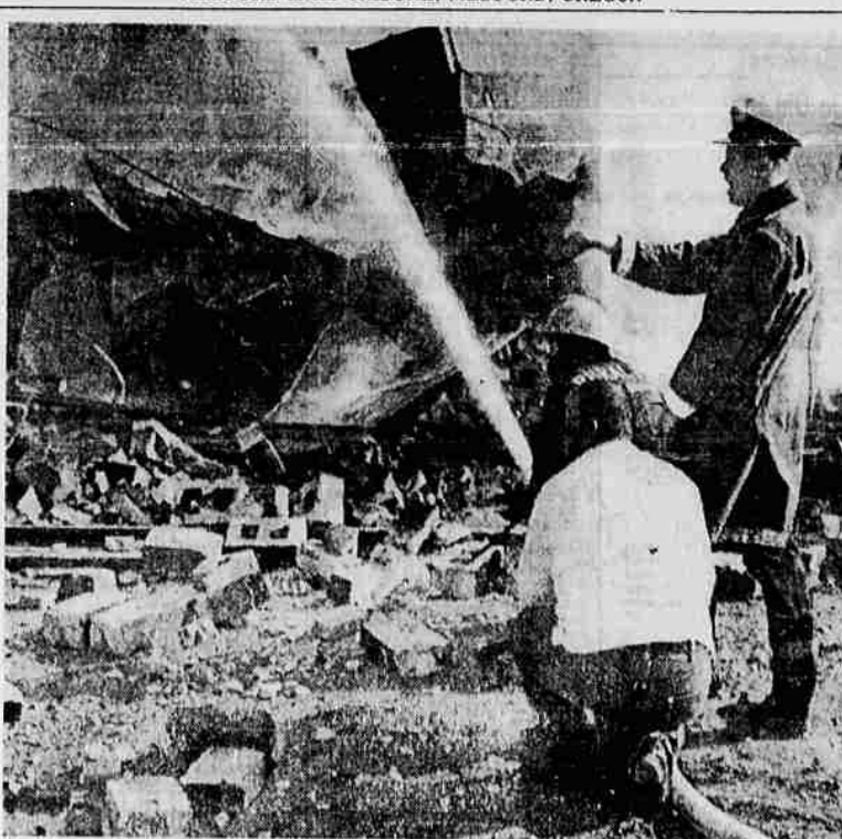
FACTORIES BURN—Fireman spray the remains of a fire which destroyed an estimated $500,000 worth of property, including the Sportcraft Trailer Manufacturing Co., and Kool-Vent Awning Co. in Tempe, Ariz. (UPI)
