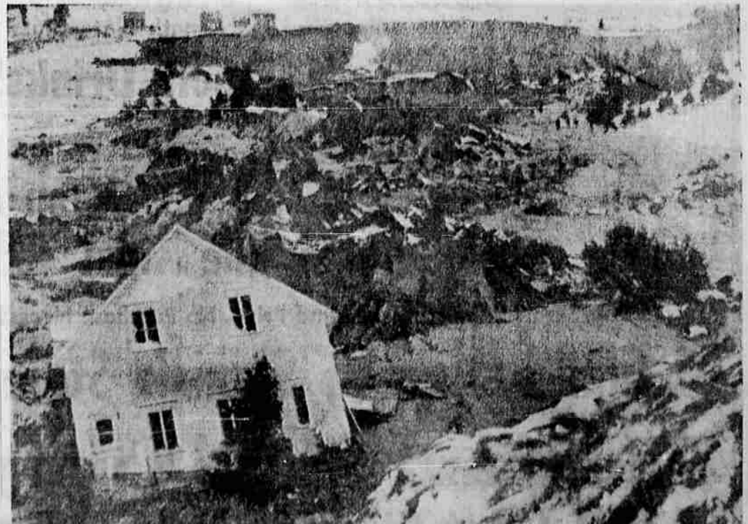
FOUR DIE IN LANDSLIDE — The above picture shows the damage caused by a series of landslides at St. Joachim de Tourelle, Que., killing four persons and injuring many others. At least six houses and a bridge were washed away into a
