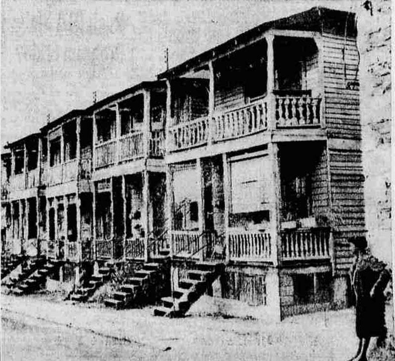
NEGRO TENEMENTS — Negroes still live in these ancient and rundown tenements on the south side of Atlanta, Ga. Understandably they want something better, and many are able to pay for something better. In many cities, though, the "something better" just isn't available. (UPI)
