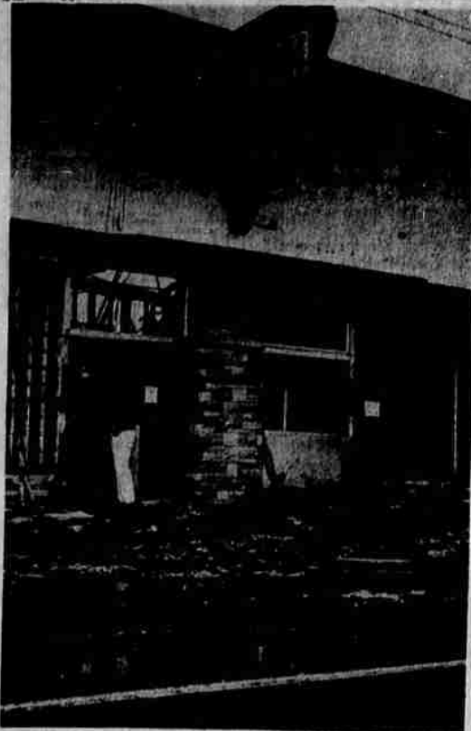
ALL THAT REMAINS — Just a shell of a building is all that remains of the Las Vegas Sun newspaper plant in Las Vegas after a faulty air conditioner exploded and set fire to the building, which houses the offices and presses, early Wednesday morning. Sun Publisher Hank Greenspan is away in Europe, but his staff is making arrangements to continue publication of the paper at another plant. (UPI)
