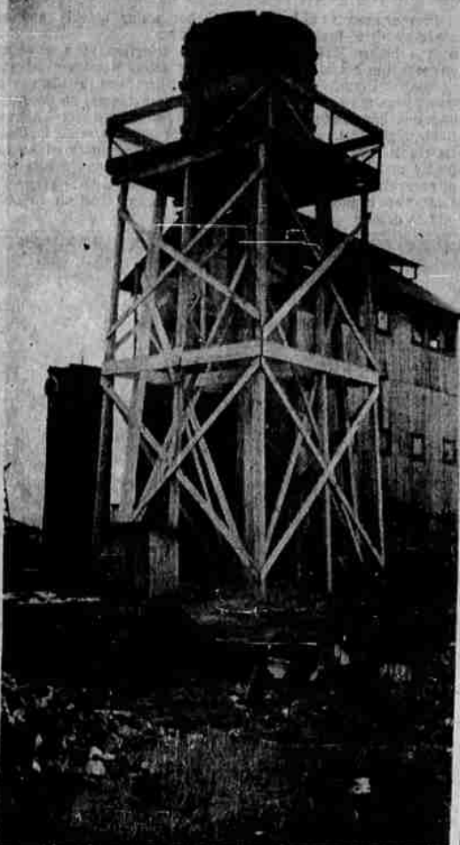
PHOENIX PLANT — This picture shows the oil-gas plant which was located about a mile north of Phoenix. It served gas to the cities of Medford, Phoenix, Talent and Ashland. The original plant, which was located at this site, brought gas to Southern Oregon in 1910. The Southern Pacific Company's "Gas Works" sign is still in place beside the railroad track at the station, which is now the site of the Steve Wilson company lumber mill.
