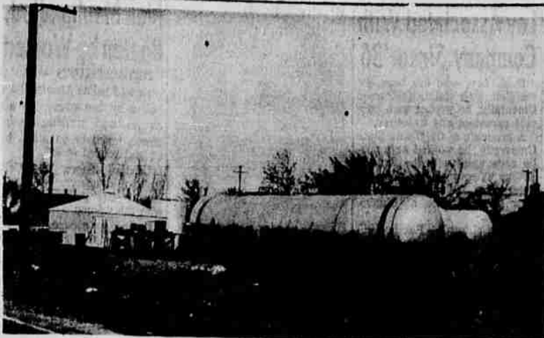
MEDFORD PLANT — The oil-gas plant near Phoenix was dismantled when district butane-air gas plants were built. The above is one of four completed in Medford during 1936. It was located at 519 N. Front St., the location of the present propane-air plant and one of the regulator stations which will provide natural gas service. The above picture was
