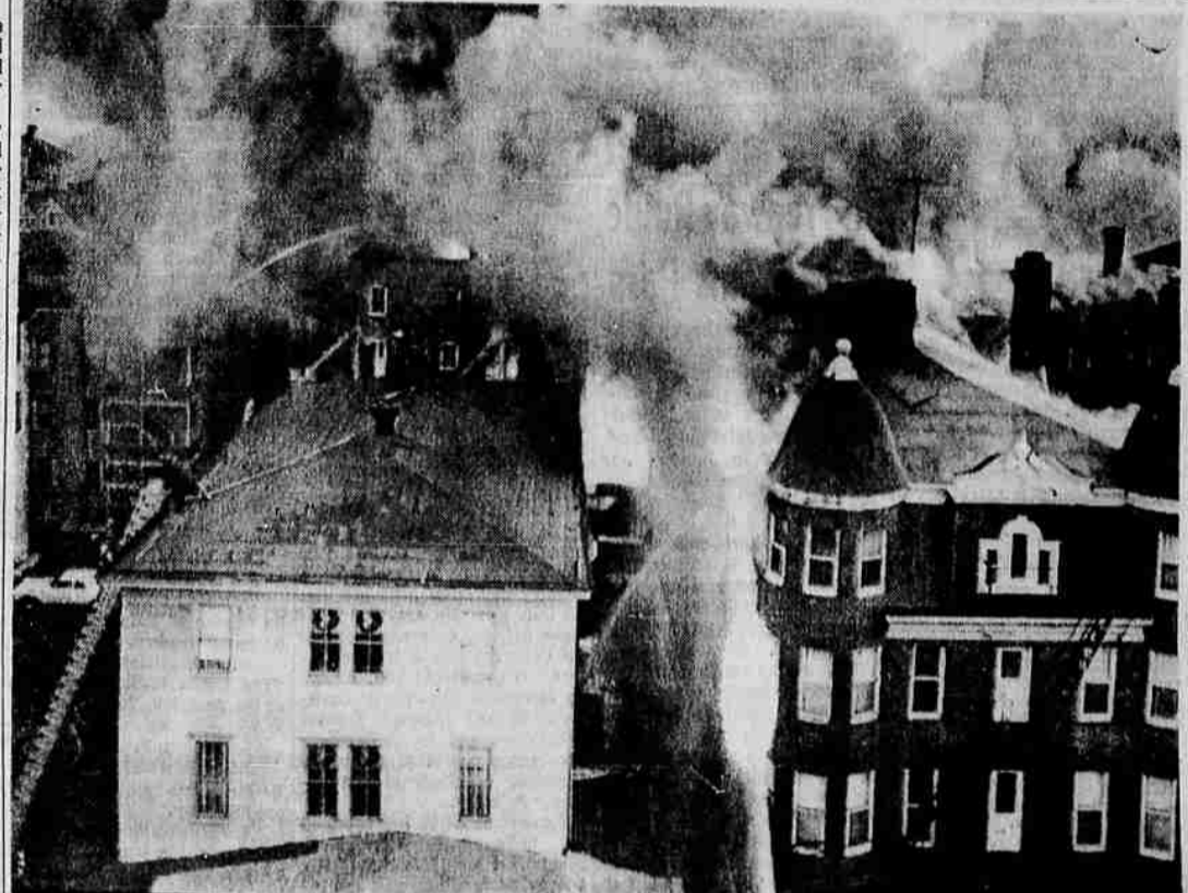
BOARDWALK HOTELS BURN — Firemen wage a heroic battle from the street and rooftops to fight a roaring general alarm fire which swept through a string of Boardwalk hotels in Atlantic City, N.J. early today. (UPI)
