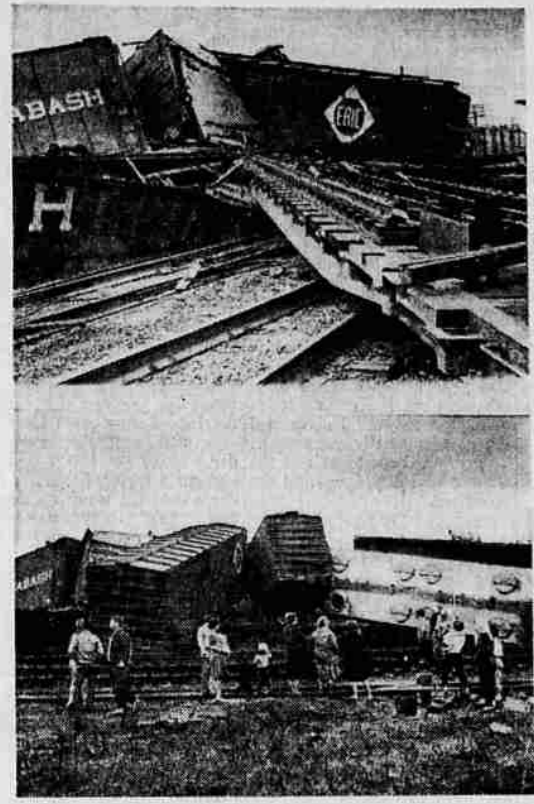
TRAIN DERAILED — Property damage ran high when 31 cars of a Frisco freight train, top photo, was derailed near Pacific, Mo. In the lower photo spectators gather as workmen make plans to clear the tracks, which were completely blocked. An unoccupied house along the tracks was damaged by the derailling cars, as was an auto parked in front of it. (UPI)
