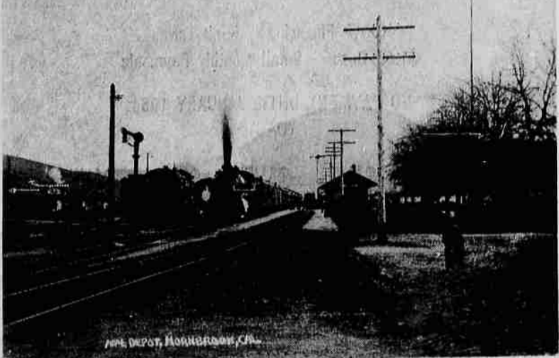
SCENE IN 1912—This old photo is taken from a post card showing the railroad depot at Hornbrook in about 1912. The T. Jones Hotel, built in 1888, was a beehive of activity in earlier days, because Hornbrook was a division point in the railroad network. As many as 32 trains a day went through.
