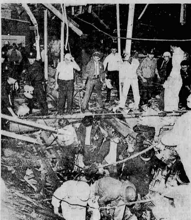
PROBE EXPLOSION—Firemen and volunteers probe giant hole in floor of drugstore in Marietta, Ga., after mystery explosion ripped crowded building Thursday. Indications were that the blast, which killed at least seven, occurred at this point near front of the building (UPI)
