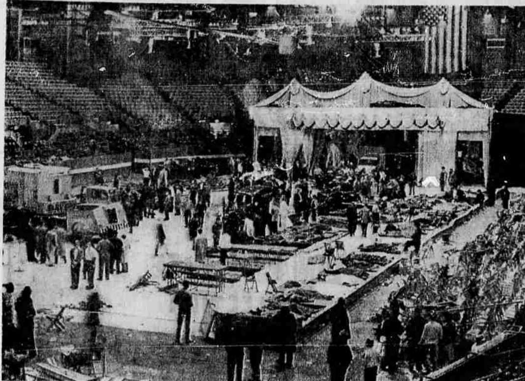
EXPLOSION AREA—This is a general view of explosion area at the Indiana State Fairgrounds Coliseum in Indianapolis last night. In background is stage where the ice show was
