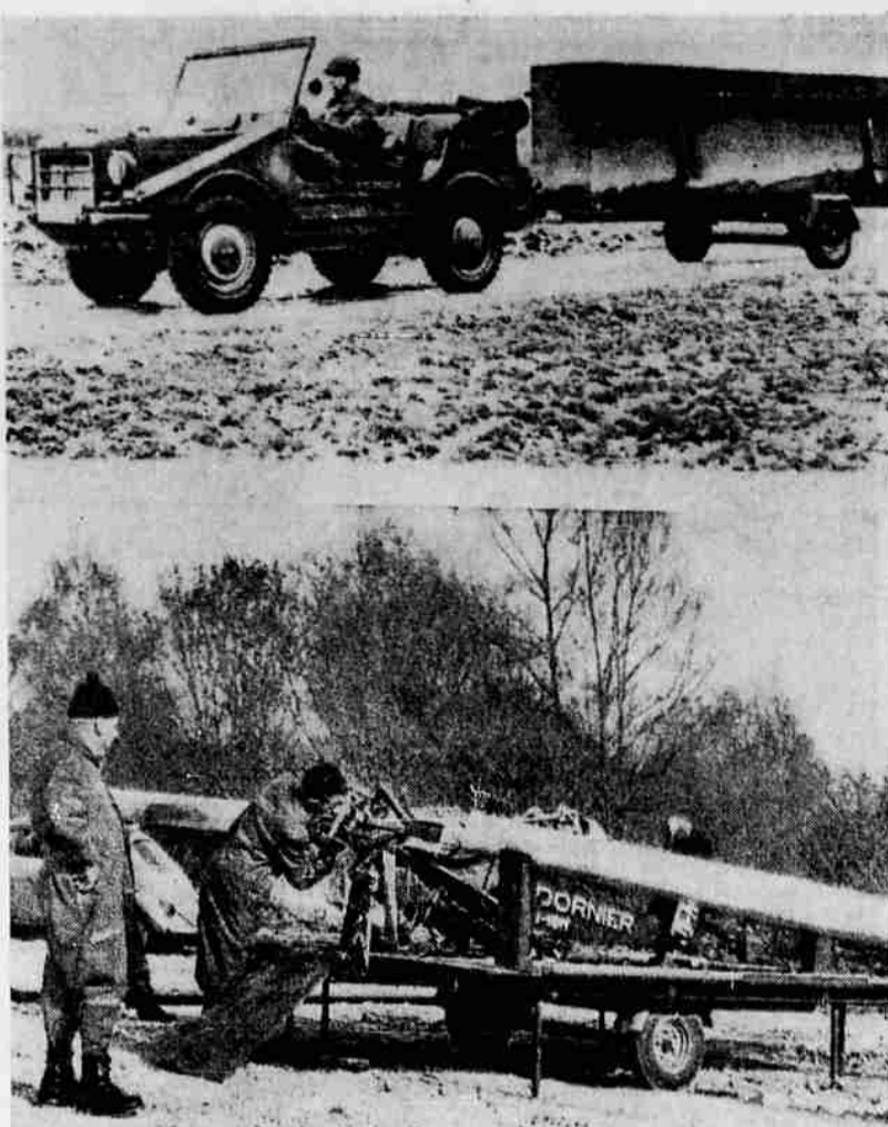
COLLAPSIBLE HELICOPTER — The first collapsible reaction-type helicopter, the Dornier DO 32, is demonstrated to officials at the Pentagon. The DO 32, a single-seat jet turbine chopper, can be folded into a box-like trailer, top photo, which serves as its takeoff and landing platform. From its folded state it can be erected and flown in less than five minutes, bottom photo. The chopper has a cruising speed of 54 knots and an operating range of 56 miles. (UPI)
