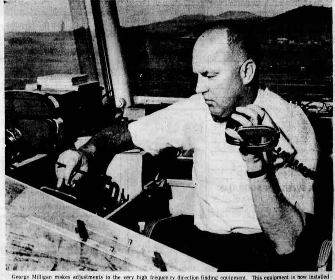
George Milligan makes adjustments to the very high frequency direction finding equipment. This equipment is now installed in only a few facilities across the nation but will be placed in approximately 400 within the next two years. It is activated by a transmitted signal from the aircraft, portrayed on a cathode ray tube, which tells the controller the direction of the aircraft in relation to the tower.
