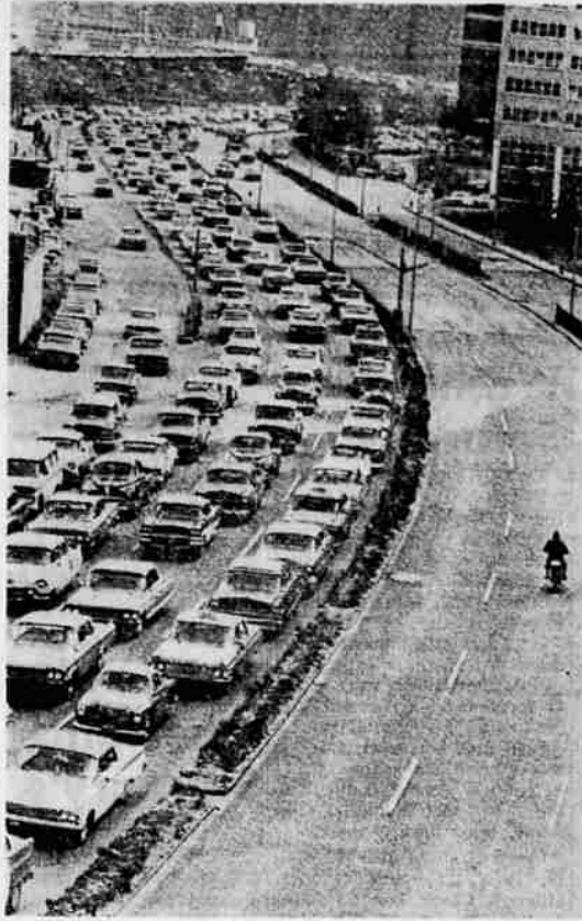
CLEAR ROAD AHEAD —A motorcyclist, right, has the southbound lane of New York's East River Drive to himself, but the northbound lane has cars lined up three deep. All northbound lanes were closed for an hour after part of the roadway collapsed, causing the massive traffic jam. (UPI)
