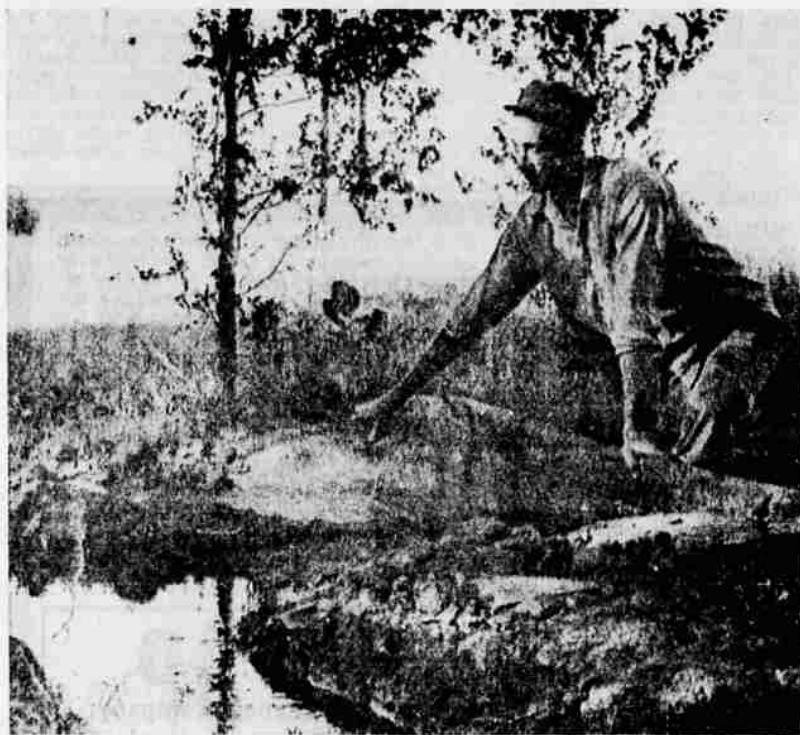
CANVAS DAM — Dennis Carter of Syracuse, Kan., places a canvas dam on an irrigation ditch to route the water to a suitable field. In the background is a dry, high plain. (UPI)
