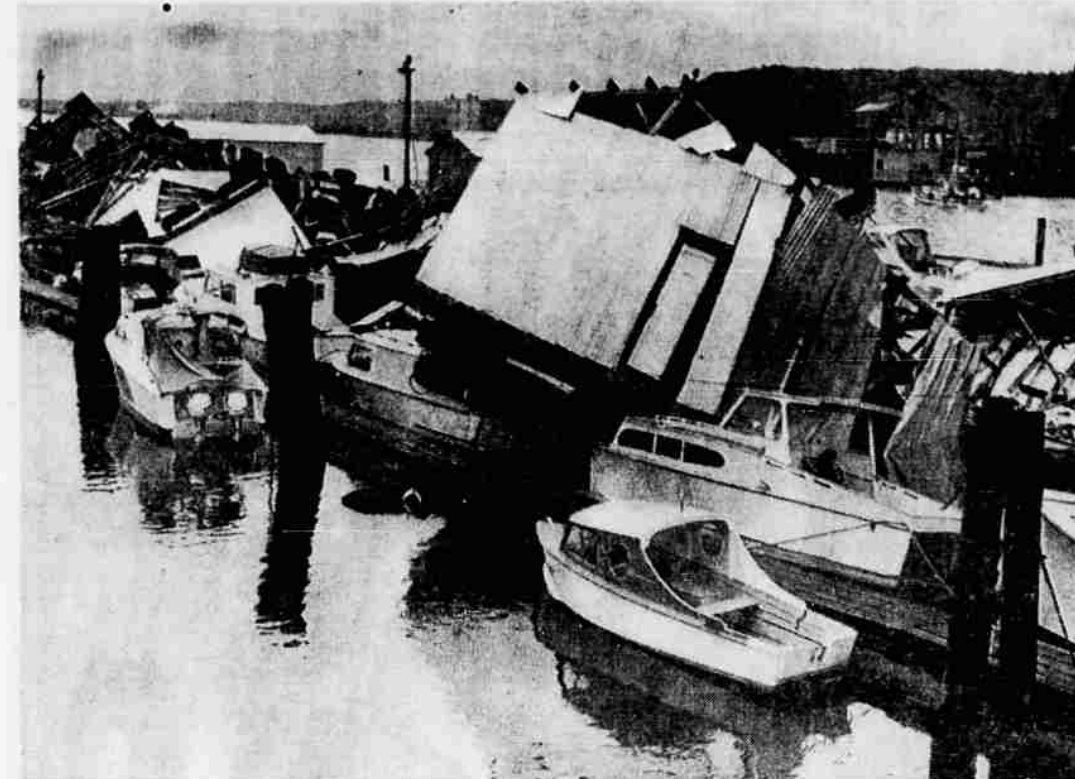
STORM DAMAGES WATERFRONT — Aftermath of Seattle's first major storm of the season, when high winds buffeted the area for several hours, is shown above. One gust of wind did most of this damage at the Anchor Marina when eight boat-houses were ripped from their foundations and were scattered among moored cabin cruisers. Damage to the marina is estimated at $15,000. (UPI)
