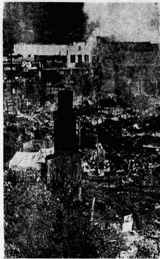
FIRE DAMAGE HEAVY — Charred and still smoking, only ashes and a few walls remain after fast-spreading flames destroyed virtually an entire block at Guerneville, Calif., on the Russian river. Unofficial damage estimates were more than $500,000. (UPI)
