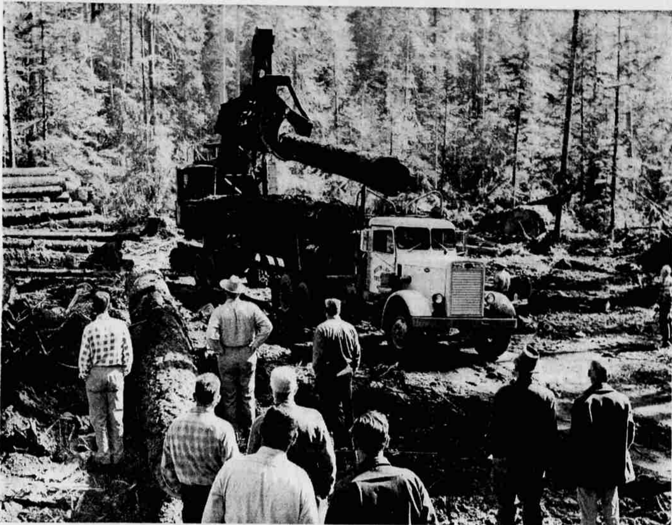
One of Medford Corporation's heel-boom loaders deftly eases a log on one of Austin King's logging trucks in the Butte Falls area. Such a rig can load a truck in 15 minutes compared to the tedious method employed formerly with stationary steam (donkey) engines, winches and booms.
