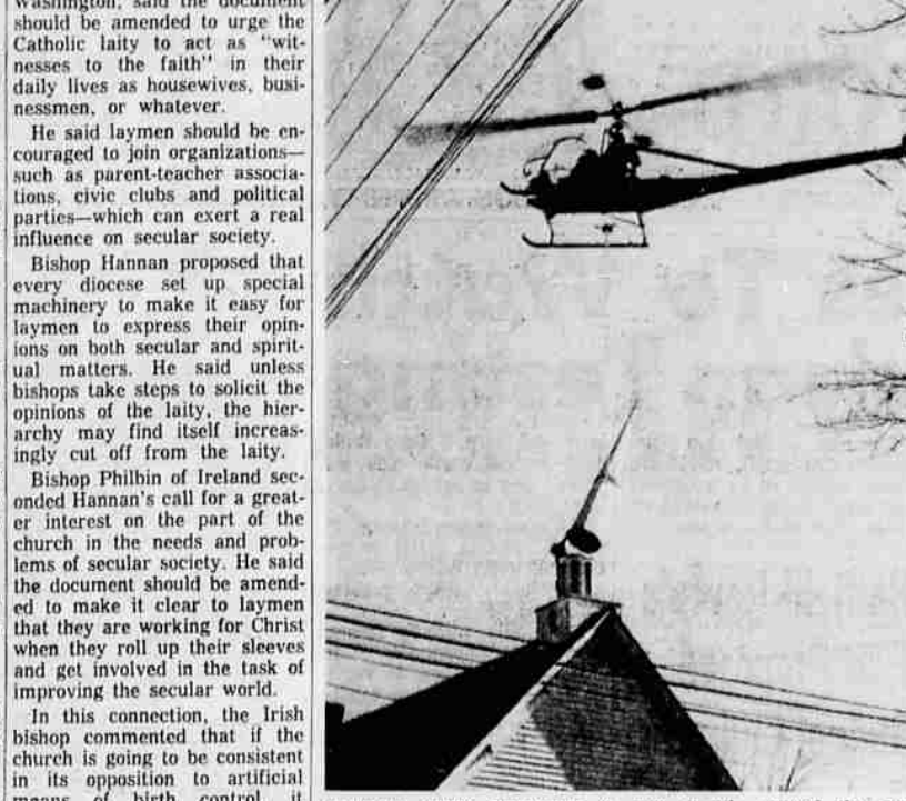
CHURCH GETS STEEPLE —A new steeple graced the roof of the Bethesda Bible Church in Ypsilanti, Mich., after a helicopter piloted by Barney Stutesman airlifted it into place. The Rev. Elton Weatherly bolted it to its base which was constructed by members of the church. The congregation stood outside to watch as the airlift operation put the finishing touches on the project. (UPI)
