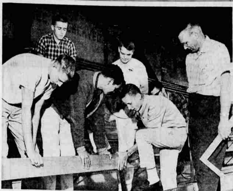
SEAT BACKS REPLACED—Students of Vern Voss's carpentry class at Medford Senior High school in a project of Thursday and Friday last week replaced the two by four-inch back rests in Sections C and D of the west grandstand of the high school stadium with two by sixes to make them more comfortable. With the lumber provided by Elk Lumber company and work donated by the students no tax money was involved in the improvement. Voss, right, supervises and holding two by six, from left, are Gary Bendickson, Ken Hackworth and
