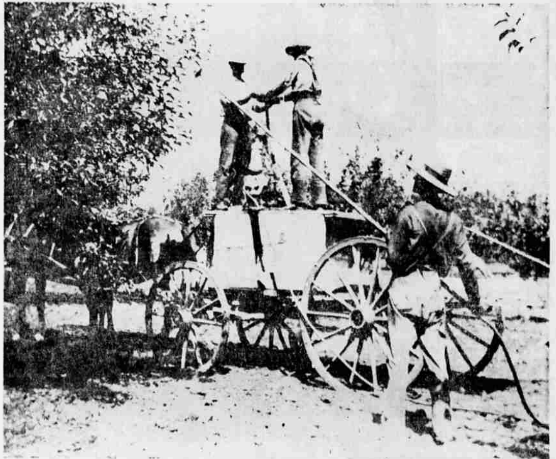
This is the first spray rig to be photographed in the Rogue River Valley, according to information given the Jacksonville Museum, where the photo is on display. The picture was taken by the late Vinton Beall. The two-man hand pump sent spray into the bamboo pole. It took three men to do the job.
