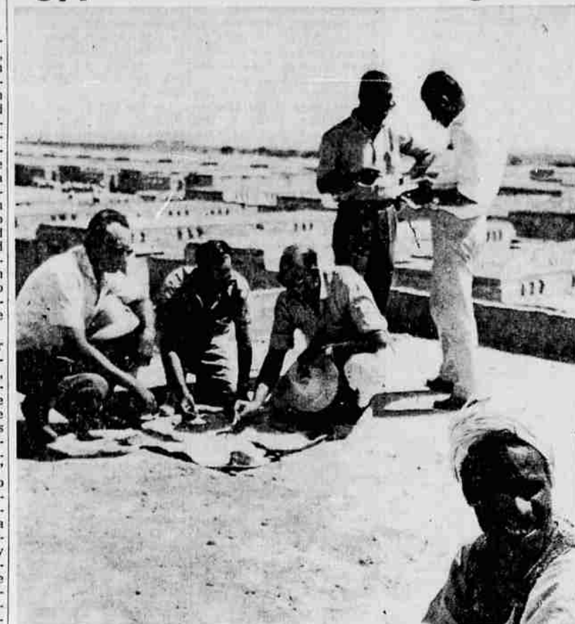
PLAN RESETTLEMENT—Engineers are shown here mapping plans for new resettlement to house Nubians displaced by the Aswan High Dam along the Nile river. In the background are partly constructed homes in the villages of Daboud, Upper Egypt. (UPI)
