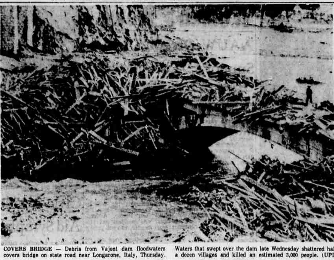
COVERS BRIDGE — Debris from Vajont dam floodwaters covers bridge on state road near Longarone, Italy, Thursday. Waters that swept over the dam late Wednesday shattered half a dozen villages and killed an estimated 3,000 people. (UPI)
