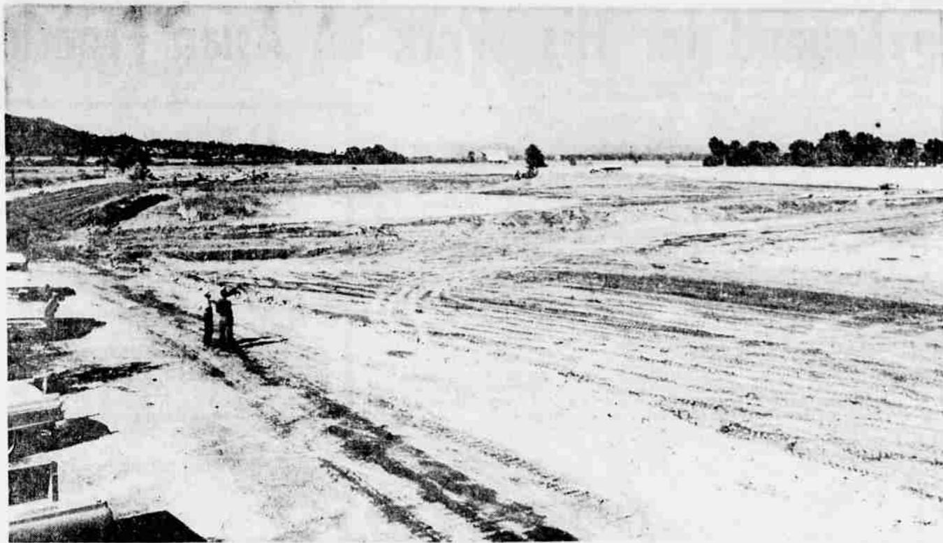
Jacksonville's sewer project will use the lagoon type of disposal system, in which sewage flows into two large open-air lagoons. Natural chemical action takes place, breaking down the sewage and eventually burning it up. The action also is said to prevent any odor from spreading. This photo shows part of the lagoons under construction on a 10-acre parcel of land located just south of the Jacksonville highway on the east side of the city.
