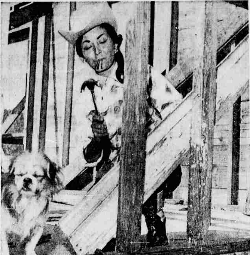
BUILDING OWN HOME — Mrs. Amanda Benavides of Austin, Texas, is an apprentice carpenter whose first project is her own home. Although her husband, a carpenter for an Austin contractor, works on the house evenings and week ends, she is at work every day "to get the job done sooner." Of her work, Mrs. Benavides says "I hit my thumb too much—sometimes I want to cry." Her dog looks as if he is expecting her to hit her thumb again. (UPI)
