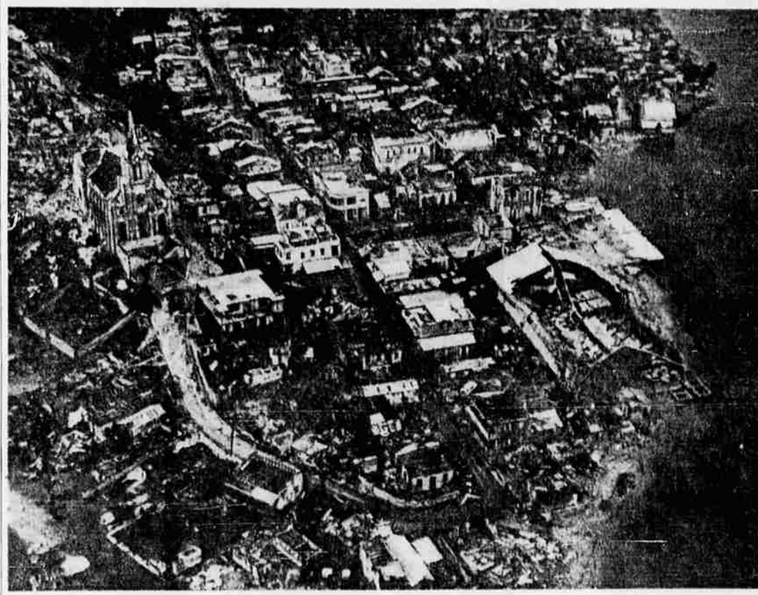
SMASHED BY FLORA — The town of Balao on Haiti's southwestern coast was smashed by hurricane Flora Friday. Whole buildings were crushed and most roofs were torn off. Oriente province in Cuba was later devastated by the storm. Direction the hurricane would take was still uncertain Saturday night, but U. S. Weather Bureau officials in Miami, Fla., warned the huge storm might move towards the mainland of the United States. (UPI)
