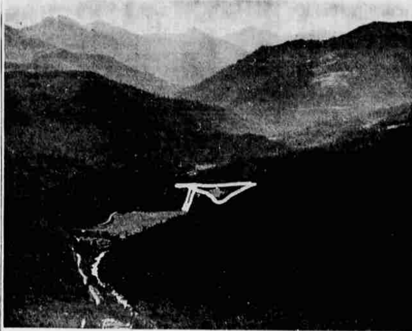
TO SERVE APPLAGATE—The Applegate reservoir, on upper Applegate river, will be operated specifically to serve the need of the Applegate valley. About 70,000 acre-feet of storage will be held behind a 230-foot dam at the site shown. The pool, extending from the damsite to a point across the Oregon-California boundary, is expected to provide large recreation, fish and wildlife benefits as well as control of Applegate river floods and additional irrigation water.
