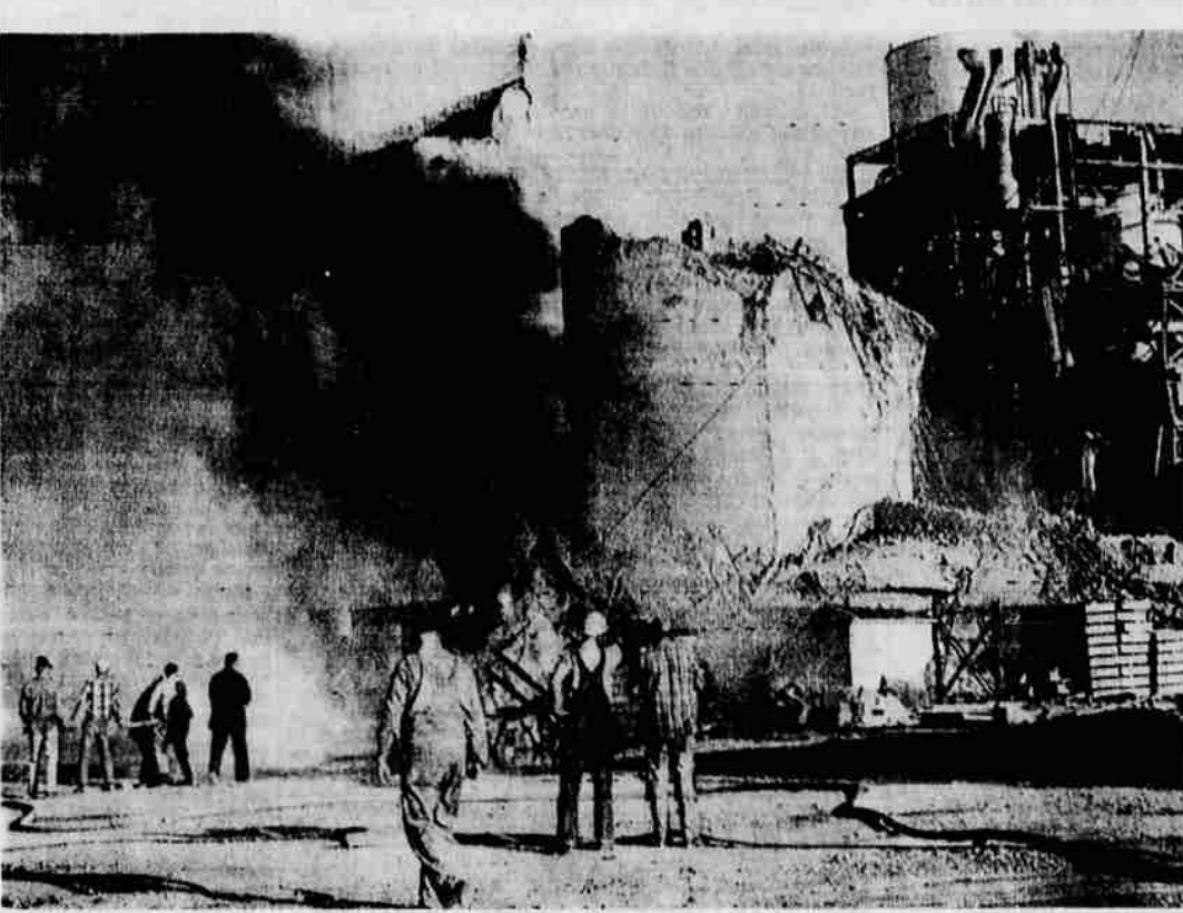
REFINERY DAMAGED — Four people were reported killed when the U and I Sugar refinery at Moses Lake, Wash., was severely damaged by an explosion and fire Wednesday. Four of the eight silos at the plant were destroyed by the blast, of unknown origin. (UPI)
