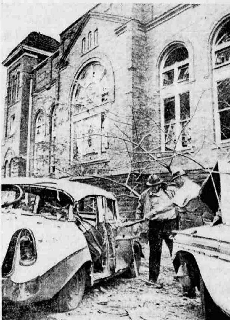
CHURCH BOMBED—A police officer points out damage to an auto outside the Sixth Avenue Baptist church in Birmingham, Ala., following a bombing Sunday which killed four persons and injured at least 12. The blownout window indicates the force of the blast. (UPI)
